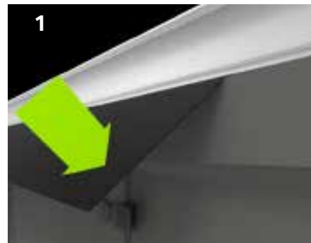
If glass roof fold the EPDM over the walling membrane.
